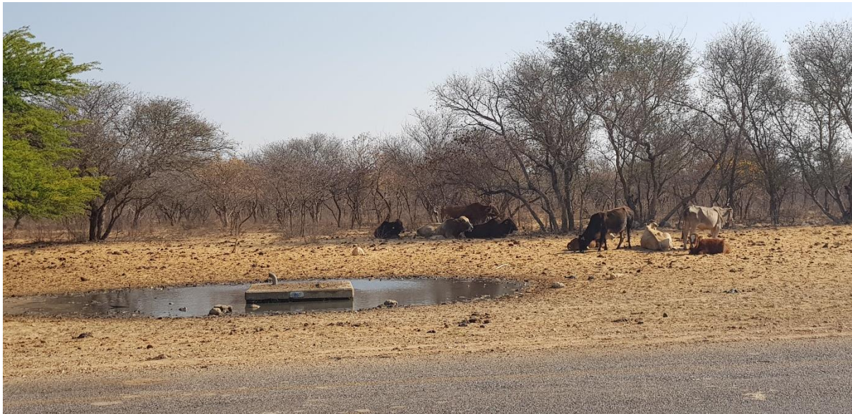
Figure 27: An example of ponding around a pressure release value on a water pipeline between Serinane and Molepolole [SOURCE: Gosiame Neo-Mahupeleng]
